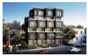
The Cabin at 45 Dovercourt is a six-storey wood structure consisting of 25 units with two floors in each. The units range in size from 895 square feet to 2,638 square feet. It is designed to be in the form of cubes stacked on top of each other. - Photo: RAW DESIGN
